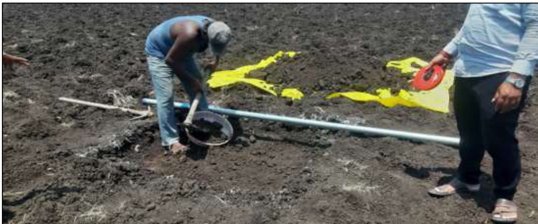
Plate 2. Digging of pit and heave of soil from pit
