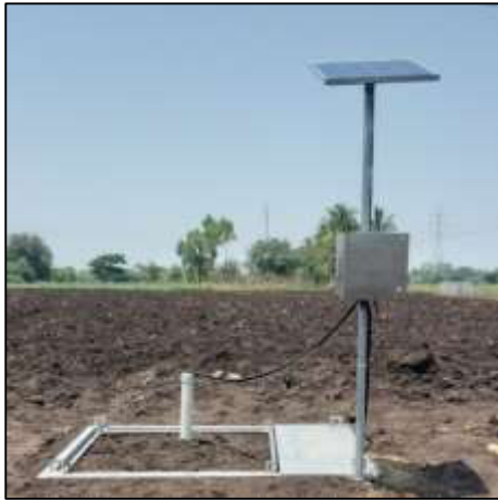
Plate 13. Final installation of Lysimeter and control panel
