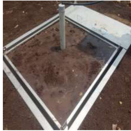
Plate 14. Saturated Lysimeter after successful installation and calibration
