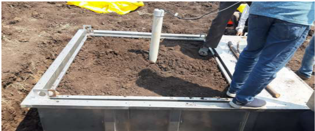
Plate 11. Completion of Soil filling in the inner tank of Lysimeter
