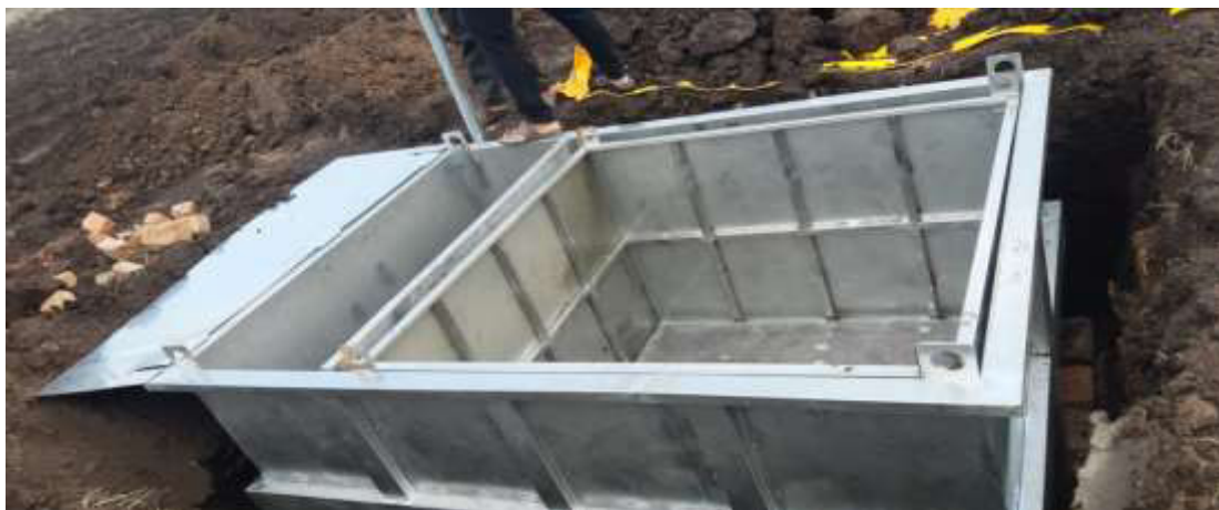
Plate 8. Lysimeter placed on the foundation in pit
