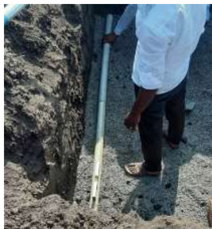
Plate 4. 1m × 1m pit from which soil was excavated layer wise to fill in inner tank of Lysimeter
