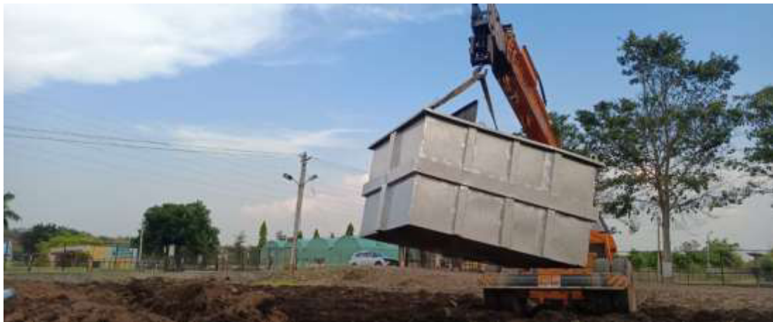
Plate7. Transportation of Lysimeter to site
