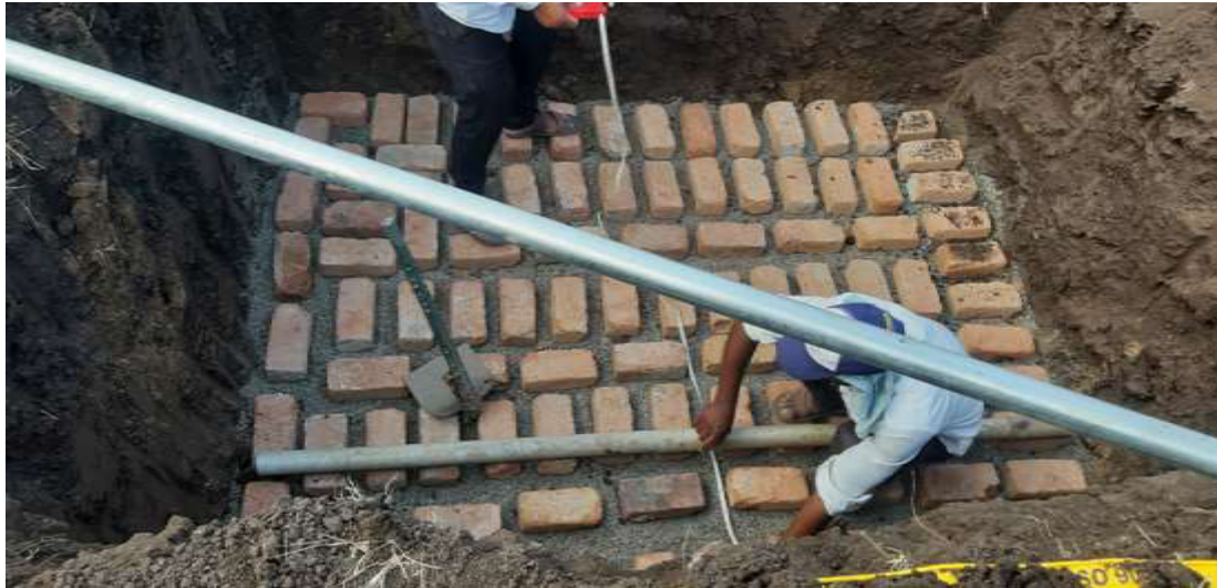
Plate6. Bricks foundation below Lysimeter as levelled platform
